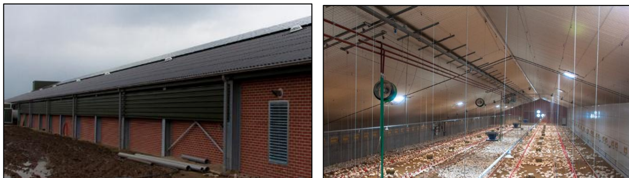
Figure 10. Fourteen solar tubes installed in two rows on the roof of a Dutch broiler barn. (a) The first image shows an external view of the broiler barn with the solar tubes installed on the roof. When this image was taken, the outdoor light intensity on this cloudy day in the Netherlands was reported as \sim 1200 lux. (b) The second image shows the inside of the broiler barn lit by the entry of natural light through the solar tubes (Source: Poultry Daylight UK).
